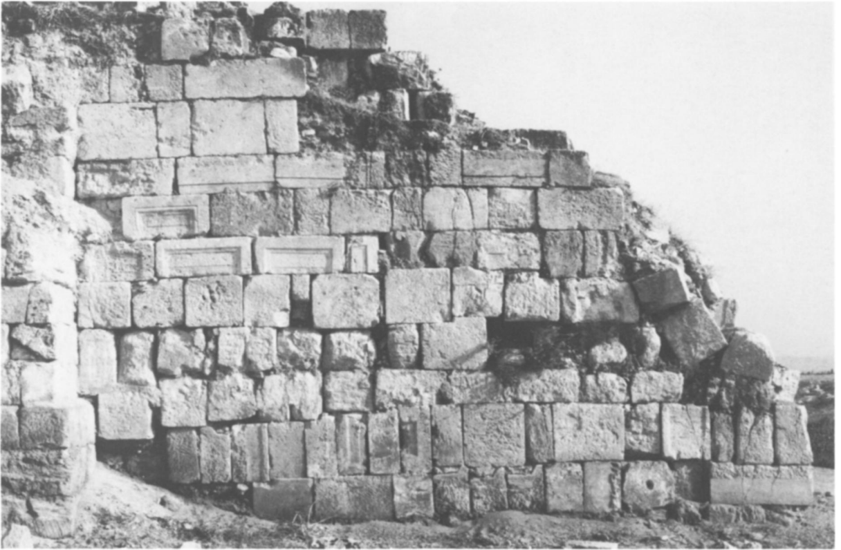
(1) SOUTHERN FACE OF TOWER XV, BEFORE DISMANTLING WORKS (1986)
